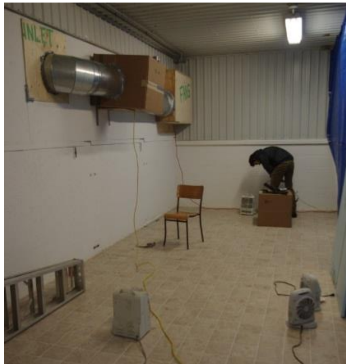
View of the prototype testing phase
