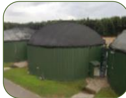
Anaerobic digester digestate
