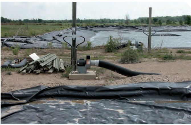
Figure 36. Tight-fitting negative pressure tarp for liquid earthen manure storage (V6).
