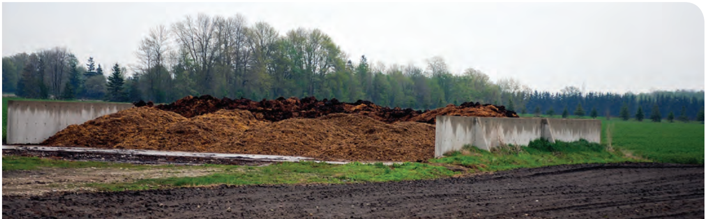
Figure 33. An outdoor, uncovered solid manure storage (V3).
