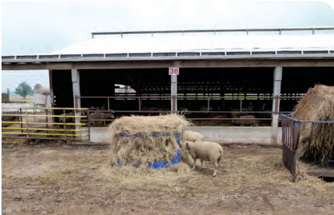
Figure 22. Exterior of a sheep barn and yard.
