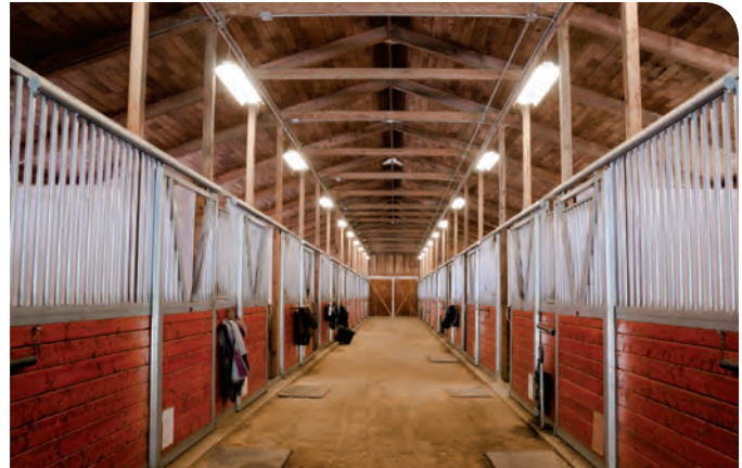
Figure 21. Interior of a horse barn.**
