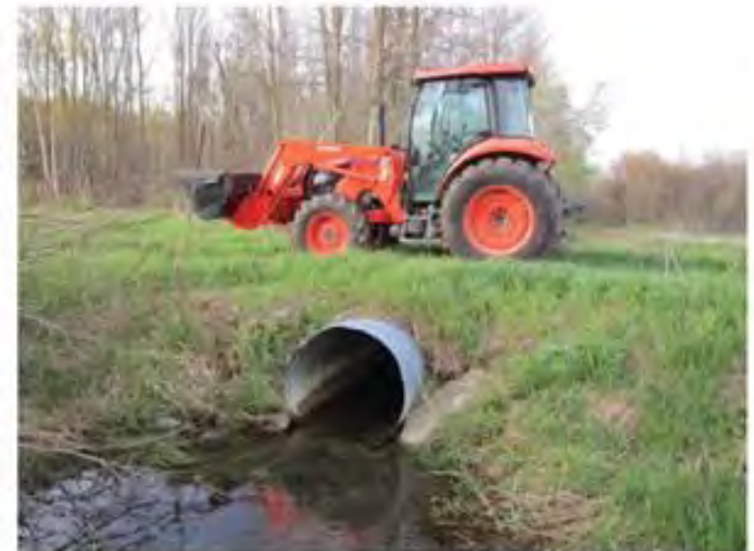
Figure B10-3. Farm equipment on a private crossing.
